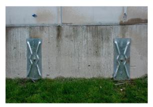
After the helical tiebacks were torqued up, tieback adapters were attached to threaded rods, the holes were patched, and wall plates installed on the exterior of the retaining wall. The wall is now permanently stabilized against further lateral displacement.
