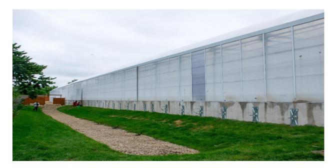
A total of 56 Class 178 Helical Tiebacks were installed to support approximately 300 linear feet of 4' tall reinforced concrete foundation wall. 10" holes were core drilled into the wall approximately 6' on center starting 3' from the corner. Leads with single 8" flight was installed and extensions to a minimum torque of 600 ft-lbs. Such that the bearing capacity was 6 kips per tieback.
