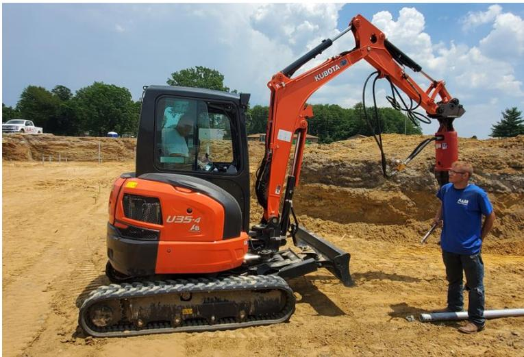
The project was completed in stages with work continuing through September of 2020. Additional work is planned as well, beyond the original 145 helical piers. The average depth per pier was 21' with the deepest piers going 35' to achieve a torque of 8,000 ft-lbs creating a bearing capacity of 72 kips per pier. With the piers in place, the footings could be poured, creating a stable foundation that will not move for the life of the home.
