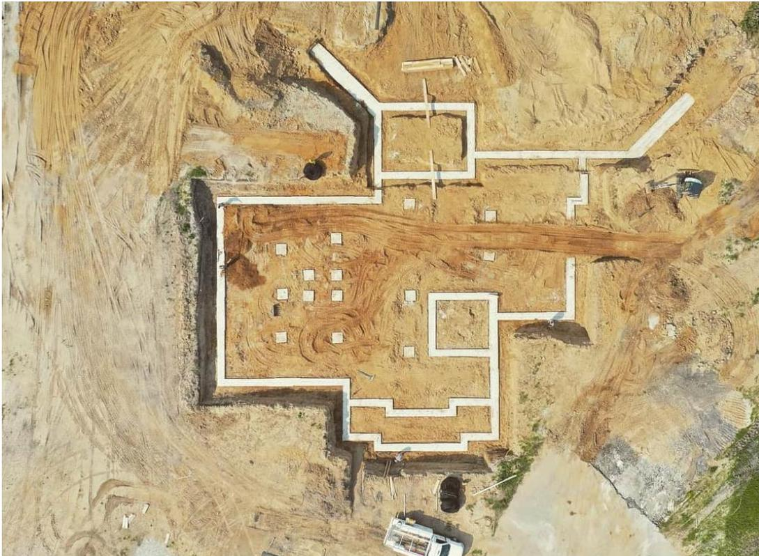
A&M Home Services was contacted by Heritage Builders regarding a new foundation to be designed for a home in Lakeville, Indiana using helical piers. SafeBasements created a set of plans which were approved for the project. The plan consisted of 145 SafeBase 2.875" OD Standard Duty Helical Piers with 10"-12"-14" flights to be used to support the footings for the home.
