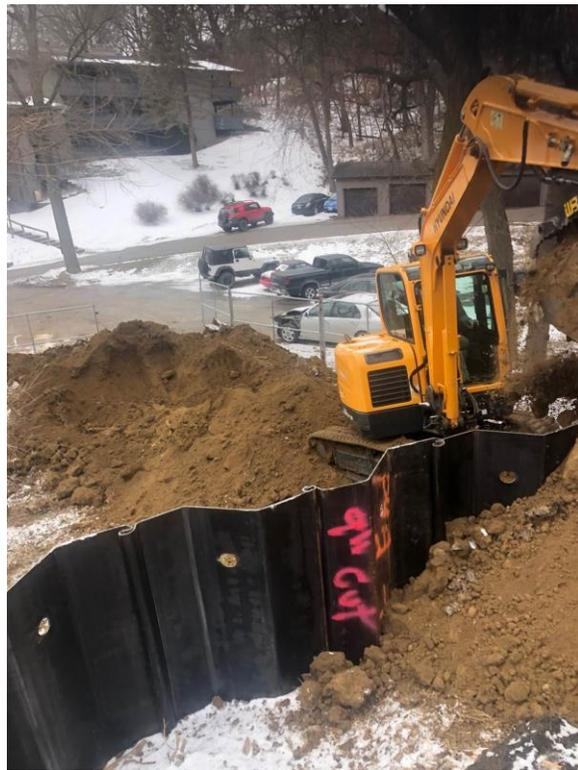
2.875" O.D. standard duty helical piers were used with tie back adapters and custom wall plates made to fit into the sections of the sheet pile wall. The project was completed in March of 2021. The new retaining wall will hold the slope stable allowing the road to be traveled safely for years to come.
