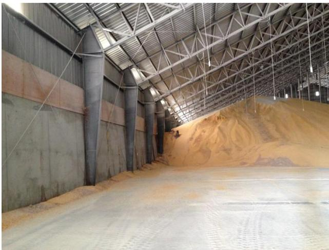
SafeBasements of Minnesota was contacted regarding movement of the walls of the grain storage building in Oakes, ND. Measurements were taken and found that the footings were settling and rotating along both of the 500' eastern and western walls. A plan was made to install SafeBase Commercial Duty Helical Piers to lift and rotate the footing back into position. The project was completed in August of 2015.
