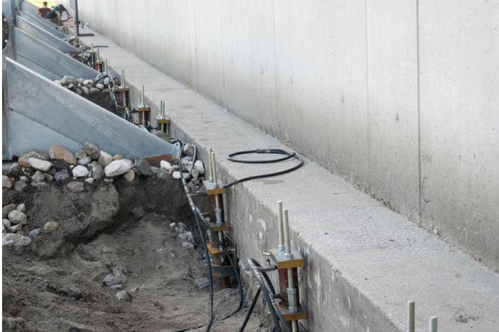
Measurements were taken along the footing, both where it meets the wall, and at the outer edge. Measurements were also taken of the lateral displacement of the wall. A correlation was found between the rotation of the wall and the footing. A plan was made to lift and rotate the wall, using 96 SafeBase 3.5" O.D. Commercial Duty Helical Piers.
