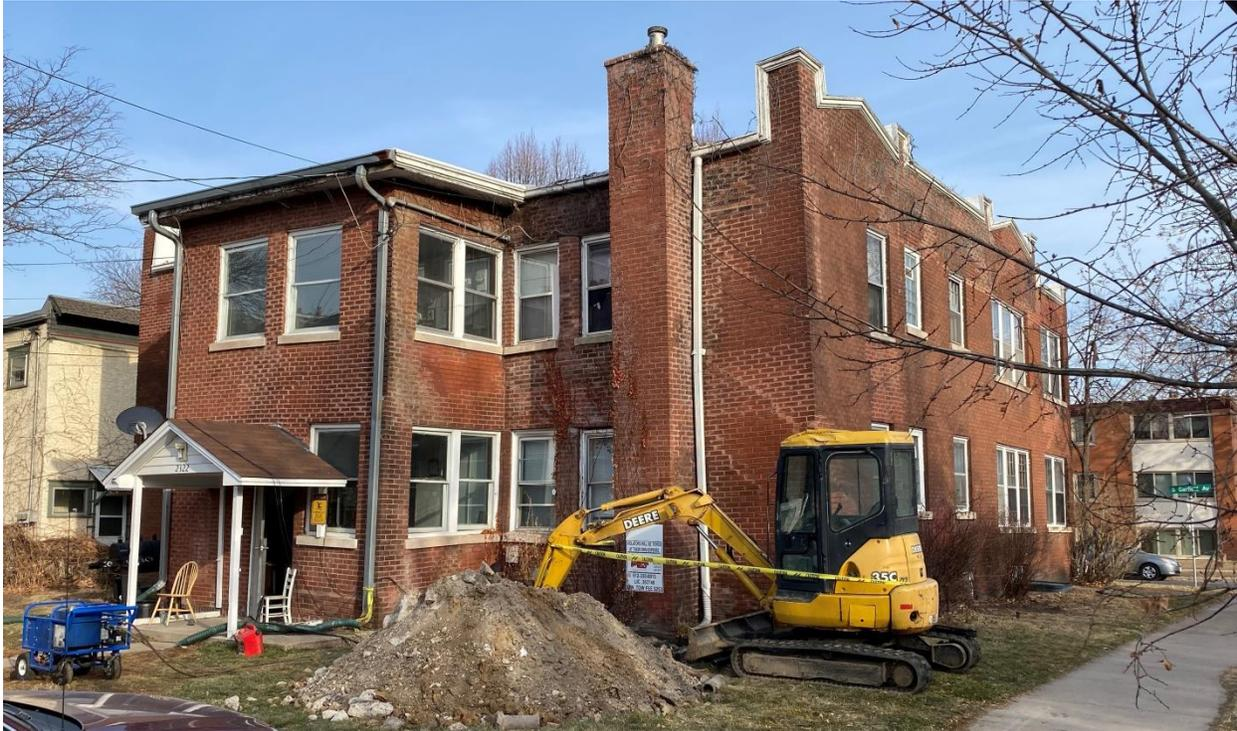
SafeBasements of Minnesota was contacted with concerns regarding sloping floors, cracks in the foundation and continual repairs needed to the brick veneer. A site visit was made and laser levels were used to take elevation measurements throughout the structure. The maximum magnitude of differential settlement was found to be 8-1/2 inches in the south west corner.
