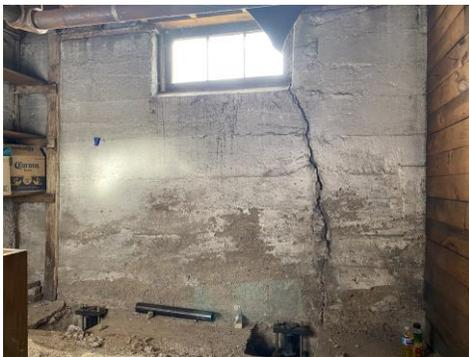
A plan was made to support the foundation with SafeBase™ 2.875" OD Standard Duty Push Piers with SafeBase™ SaberTooth™ Bracket Assemblies. A total of 22 Push Piers were installed
