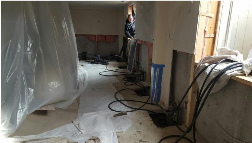
A full recovery of the 3" settlement was achieved during the lift, bringing the house and garage back to level. A pressure of approximately 3500 psi was required to lift the house and surrounding soil, which corresponds to approximately 34 kips per pier lifting force.
