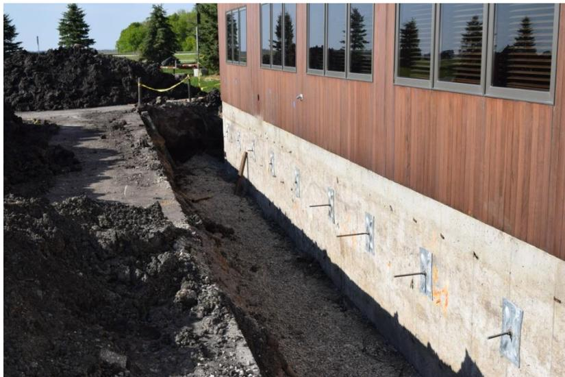
Multiple storms occurred during installation requiring dewatering of the trench, as can be seen in the photos above.
