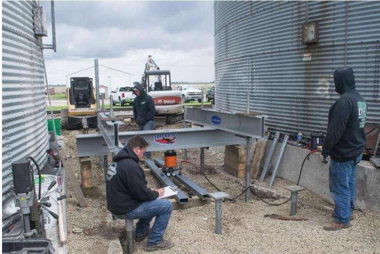
An eleventh pier was installed in the center of the group of piers in order to perform a load test. Both a tension and compression test were performed verifying the capacity achieved was acceptable for the requirements of the project. The piers were installed to depths ranging from 40 to 50 feet.
