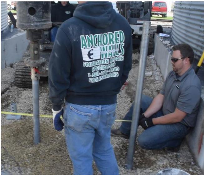
Anchored Walls was contacted by Raker Rhodes Industrial regarding a new foundation to be designed for a tower in Garner, Iowa using helical piers. SafeBasements created a set of plans which were approved for the project. The plan consisted of ten SafeBase 2.875" OD Standard Duty Helical Piers to be poured into an approximately two foot thick reinforced concrete slab. The project started on May 22<sup>nd</sup>, 2017 and was completed in two days.
