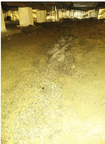
Michigan Basements was contacted by the Genesee Intermediate School District regarding water intrusion and moisture issues in the crawl space under the school. A proposal was made to fully encapsulate the crawl space, and install a full perimeter interior drainage system with multiple sump pits that would discharge the water into the storm sewer.
