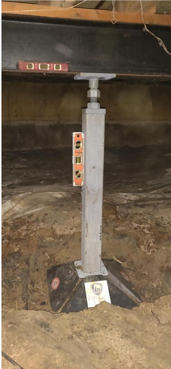
With the SafeBase™ Crawl Space Stabilizers and LightFoot™ Footings installed, the homes floor will be level and stabilized for years to come!
