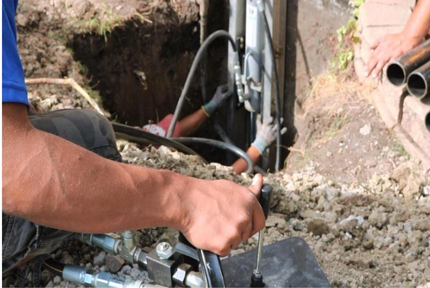
SafeBase 2.875" Standard Duty Push Piers were installed on both the interior and exterior of the home, 11 on the interior and 3 on the exterior. The piers were installed to depths ranging from 34 to 52 feet, with an average depth of 42 feet.
