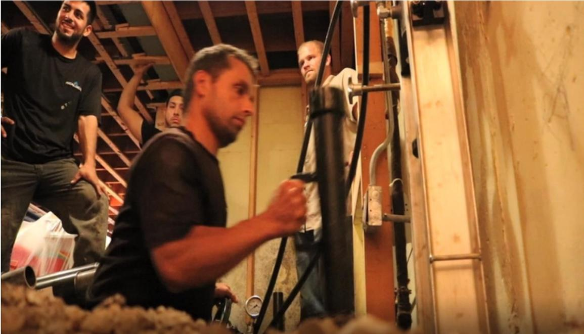
The RealSeal was contacted regarding concerns of cracks in foundation walls that would re-open each year after being repaired, allowing water to enter the home. It was found that the underlying issue of the cracks was a settling foundation. A plan was made to underpin the foundation with SafeBase™ Push Piers. Due to recent remodeling, including new windows, the decision was made to stabilize the foundation and not lift it back to level.
