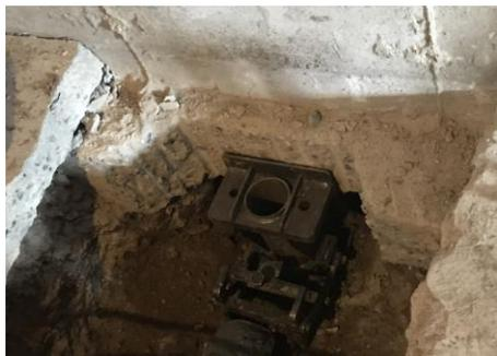
Rhino Foundation Systems was contacted by a property manager with concerns of settlement shown by cracking stucco and sheet rock. A plan was made to stabilize the foundation using SafeBase Push Piers.
