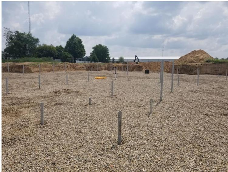
A decision was made to raise the grade throughout the whole home to keep the footings out of the water table. Six inches of #8 aggregate was then added to the base. The piers were installed to depths ranging from 14 to 21 feet at a torque of approximately 7,400 ft-lbs per pier, resulting in the piers having an ultimate capacity of 66.7 kips per pier. The foundation will now be safe to support the home for generations to come.
