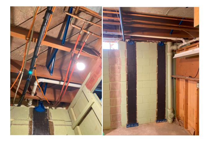
All areas that were being repaired had floor joists parallel to the wall where the top of wall restraint was to be installed. In some areas the traditional angle bracket was attached to lumber attached to the bottom of the joists with blocking or diagonal bracing installed in each joist bay. In other areas this would not be possible without moving pipes or other obstructions.
