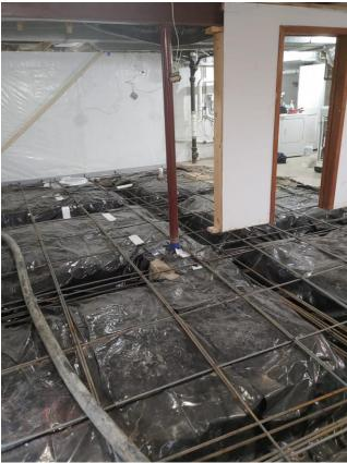
SafeBasement of Minnesota re-evaluated the situation and came up with a plan to fix the floor permanently. Approximately half of the basement floor was to be removed and replaced with a new engineered floor supported by SafeBase Helical Piers.
