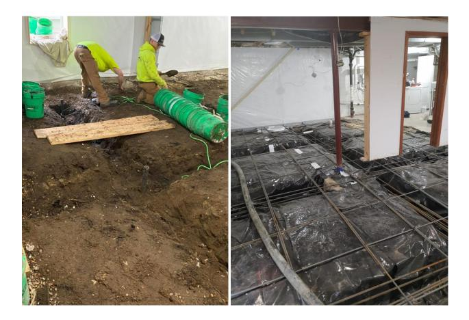
SafeBasements of Minnesota re-evaluated the situation and came up with a plan to fix the floor permanently. Approximately half of the basement floor was to be removed and replaced with a new engineered floor supported by SafeBasements Helical Piers.
